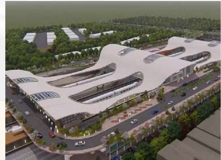
Delhi Cantonment Railway Station Redevelopment Project
